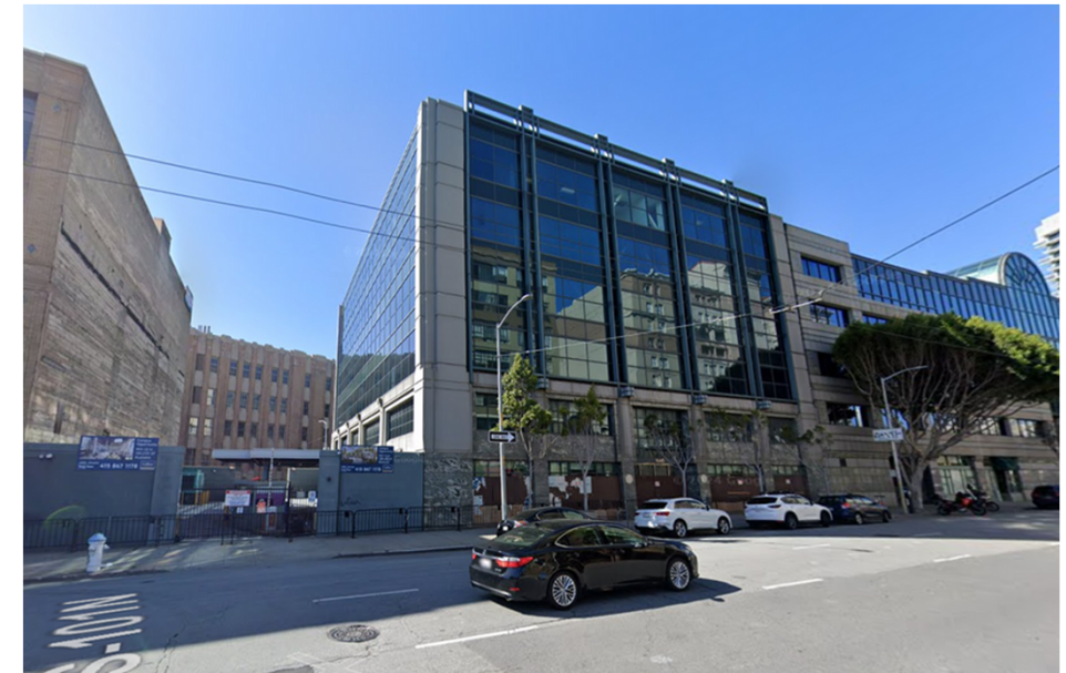
Mission Street — lobbies for MHSC and City Clinic elevators.
